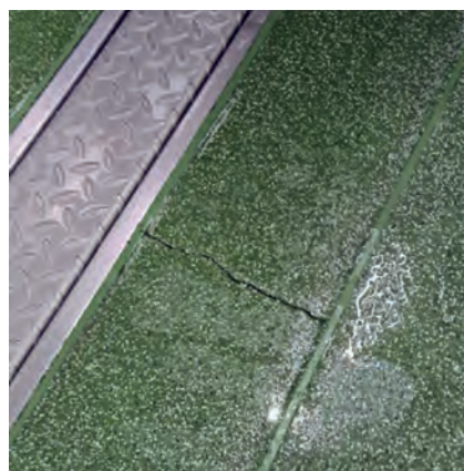
Floor area after conventional caustic hypo clean
